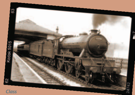
Class D49/2 No. 62751 'The Albrighton' waits to depart with the 2-55 p.m. stopping train to Hull in May 1949. The D49s were the most commonly used locomotives on local passenger services during the 1940s and 1950s. They were gradually replaced during the mid to late 1950s by diesel multiple units. Credit to P.Ward
